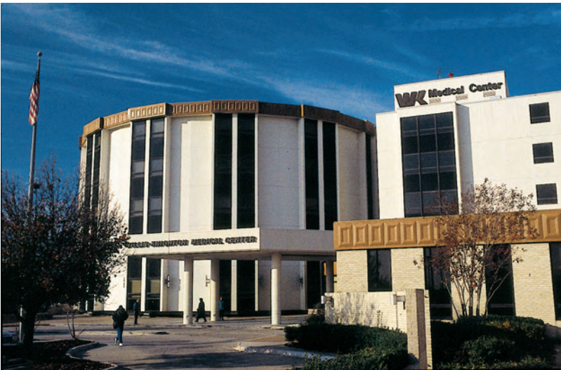
At the Willis Knighton hospital, a Munters MDAire system allows eight Surgeons to simultaneously set different OR's to the exact temperature and humidity needed for each procedure.
